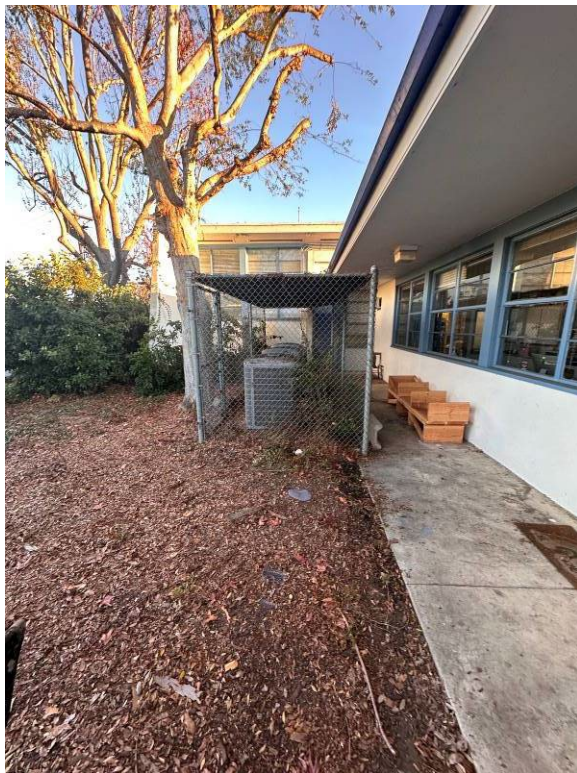
Condensing units on grade in chain-link enclosure.
