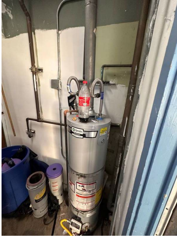
Gas-fired atmospheric tank type water heater in mechanical room.
