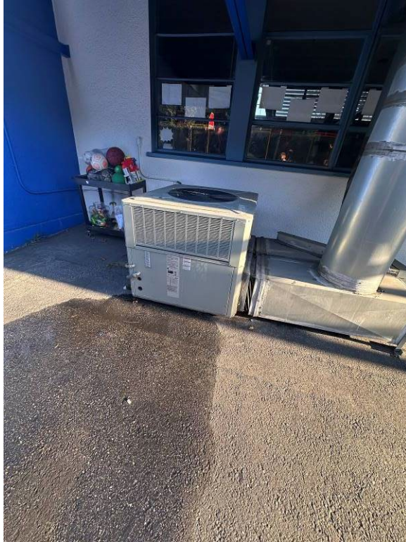
Ground mounted packaged heat pump unit serving classroom.
