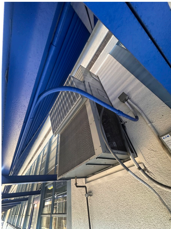
Wall mounted heat pump unit serving classroom.
