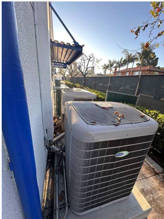
Typical ground mounted condensing unit.
