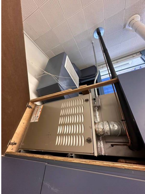
Typical classroom furnace with DX cooling coil located in casework.
