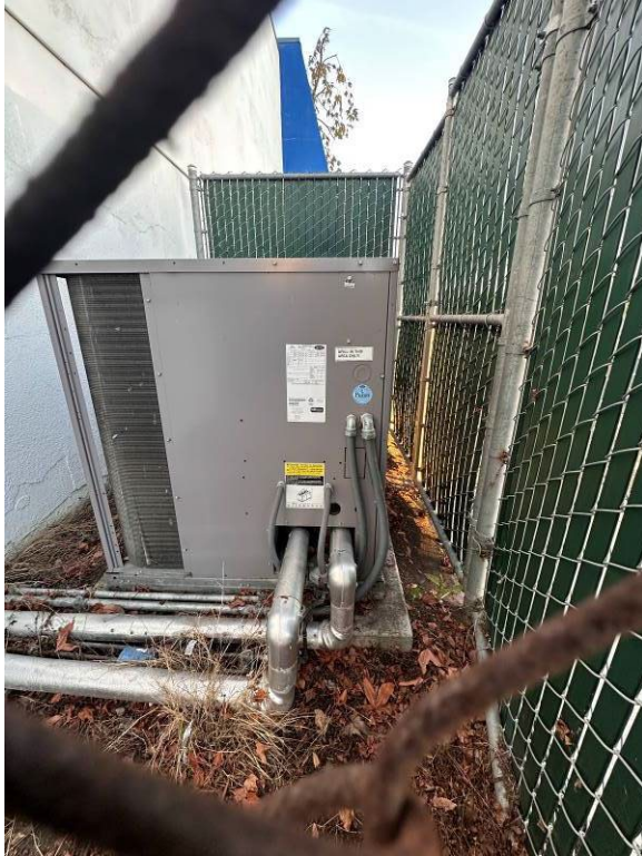
Condensing unit on grade in chain-link enclosure serving multipurpose building.
