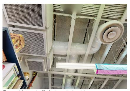
Exposed ductwork with duct mounted registers.
