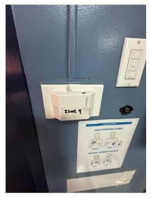
Typical Alerton zone temperature sensor connected to EMS.
