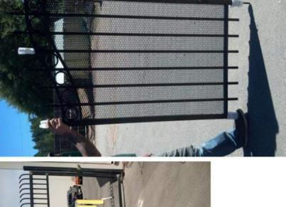
IRON ORNAMENTAL FENCING WITH WELDED MESH BACKING (THIS IS THE STYLE WE'VE RECEIVED QUOTES FOR)
