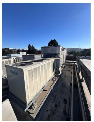
Typical condensing unit on roof serving multizone unit.
